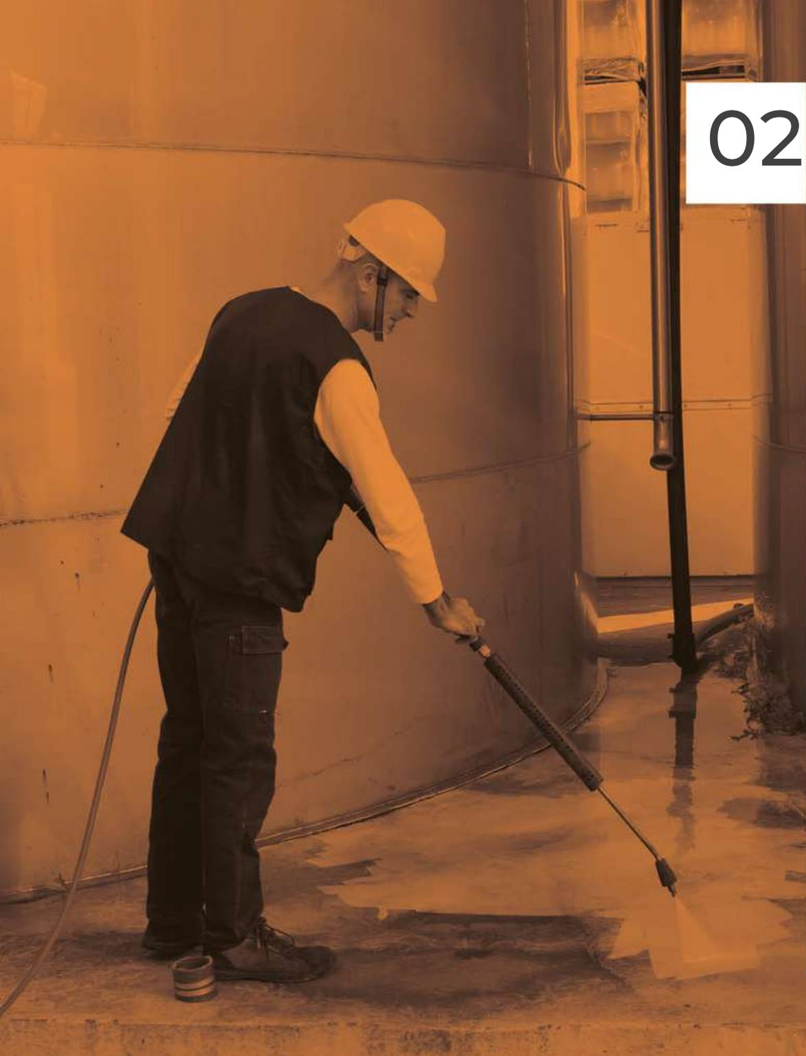
A worker wearing a white hard hat and a dark vest over a light-colored long-sleeved shirt is using a high-pressure water spray gun to clean a large, cylindrical industrial tank. The scene is illuminated with a warm, orange light, creating a monochromatic effect. The worker is positioned on the left side of the frame, facing right, and is actively spraying the tank's surface. The tank has a vertical pipe or ladder structure on its side. The overall atmosphere is industrial and focused.
